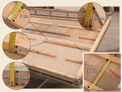
pitch width 19.8 ML:, subtract 47 cm from this width for the package on the right side of the pitch (made of DCS + the lateral closing coppo-tile) subtract another 47 cm. for the left pitch, remain 18,86 ML. each DCS occupy a space of 0,37ml: included the toleration so 51 DCS are needed for width of the pitch.
