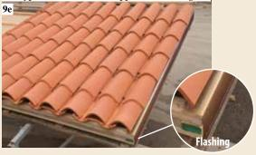
10 - We recommend to put the ventilationcoppi-tiles instead of coppi-tiles by using the spaces in the DCS.
