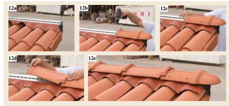
12 - Attach the laths holders needed to assemble the ventilated under ridge. This concludes the laying by placing the ridges on the under-ridge and fasten them with aluminum hooks (code 090105). If provided install the finals on the ends of the ridge line.
