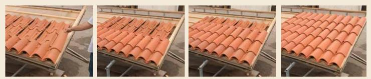
8 - Proceed posing the 45 cm coppi-tiles by laying them on the molded profiles and the clamps present in the DCS will lock the coppo-tile preventing it from slipping. After which pose another line of DCS and then cover with the 45 coppi-tiles. Continue placing alternately DCS first and then the 45 coppi-tiles.
